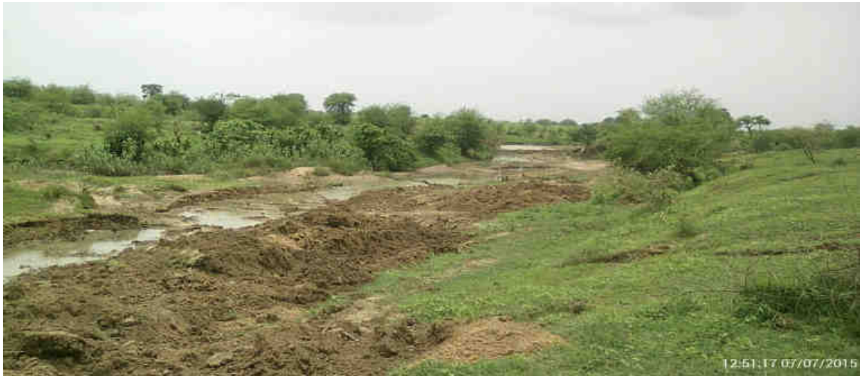
De-silting and widening of Erai River
