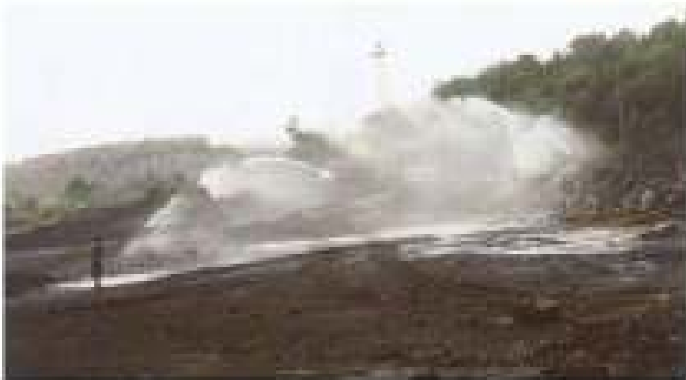
Fixed Sprinklers at Coal Stockyard
