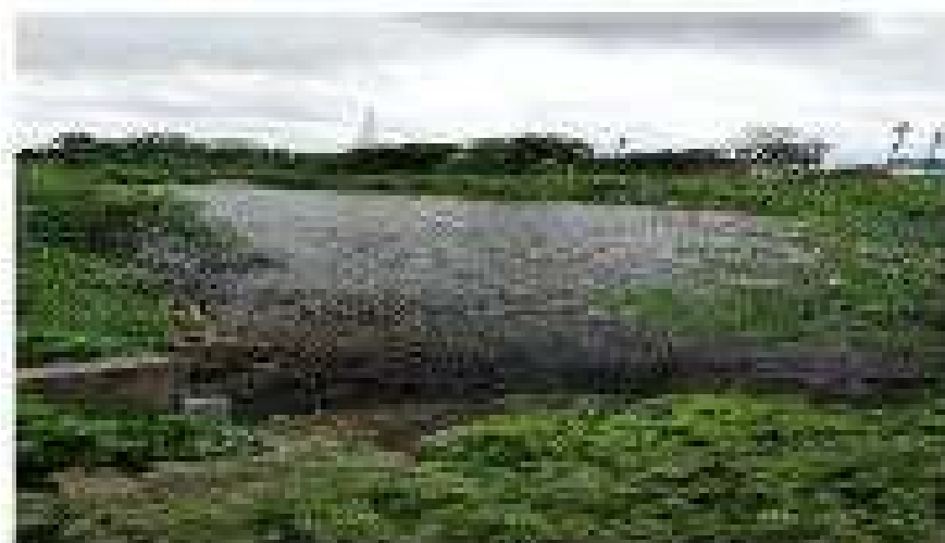
ARTIFICIAL RECHARGE POND NEAR NEW MAJRI UG COAL STOCKYARD (DIMENSION-88 m x 18 m x 1.2 m)
