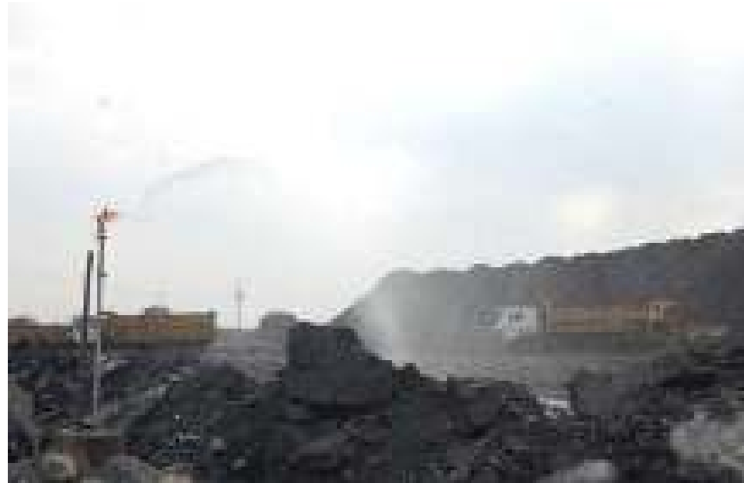
Fixed Water Sprinklers at Coal Stockyard
